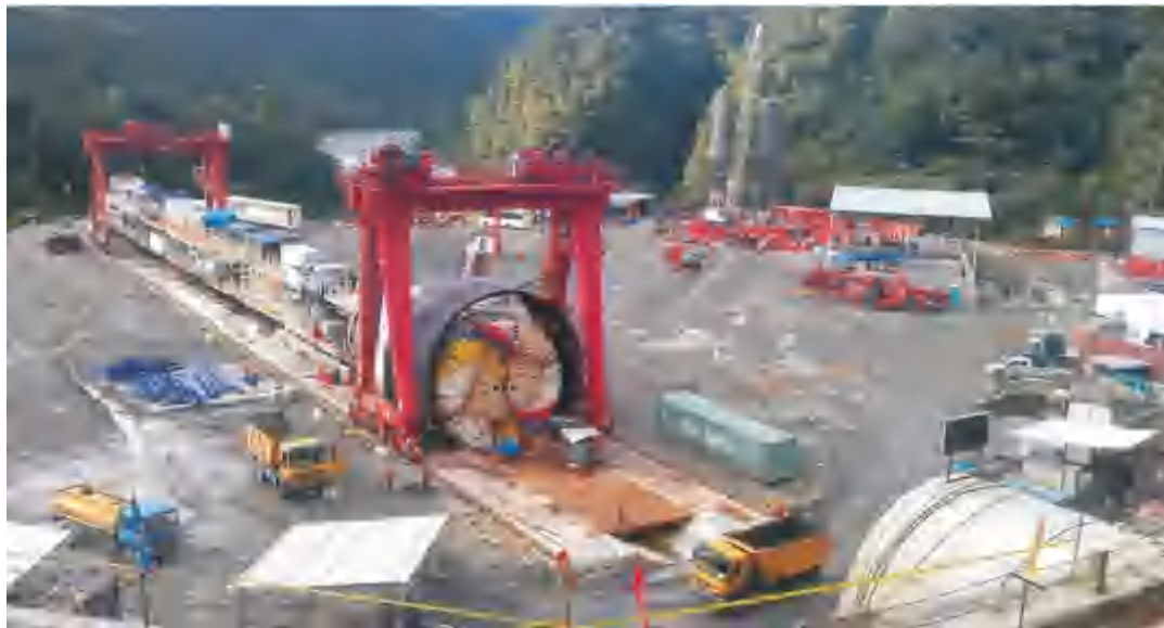
TBM组装调试
